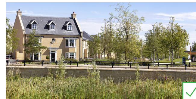
Attenuation basins can provide attractive linear features alongside major transport routes
