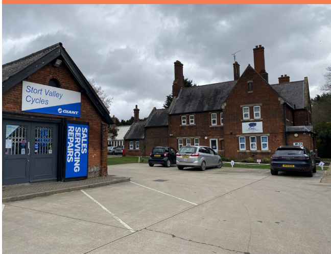
4. View looking towards the existing buildings within Village 1.
